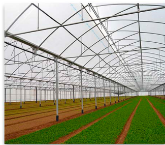
MURCIA (Spain) Invernadero Multitúnel Gótico Multi-tunnel Gothic Greenhouses 15.400 m 2
